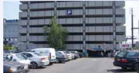
Le parking silo
